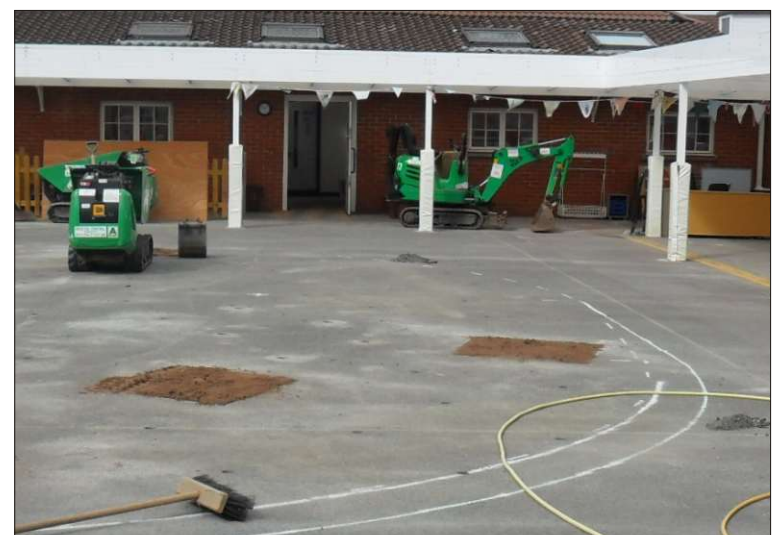
Construct on site - carpets and surfaces protected, workers compound secured, site kept tidy on a daily basis. Appropriate machinery for the job - small enough to drive through the corridors. August 2011
