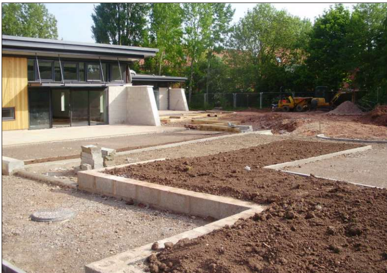
The changes in level were accommodated in a series of slopes, banks and small walls rather than a single big wall. May 2010
