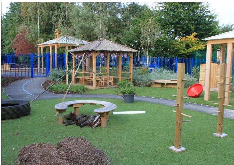
Gillingstool Nursery garden at the end of defects liability - lots of activities for the children. Snags and plant failures identified. September 2011
