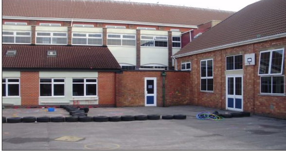
2010: Existing Foundation Stage playground
